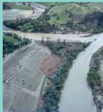
Above: Dartmoor River showing flood damage to the flats... and no bridge. Left: Sodden hangars at Bridge Pa aerodrome.
